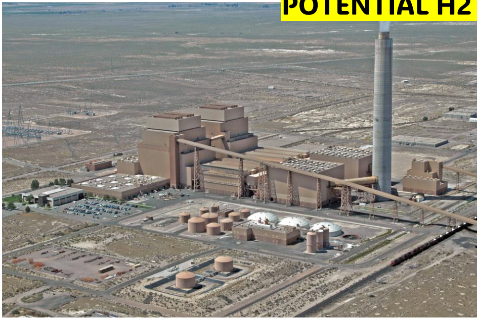
HYDROGEN BURING POWER PLANT
